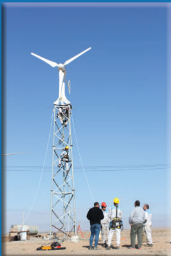
Installation of 5 kW- off grid wind turbine
